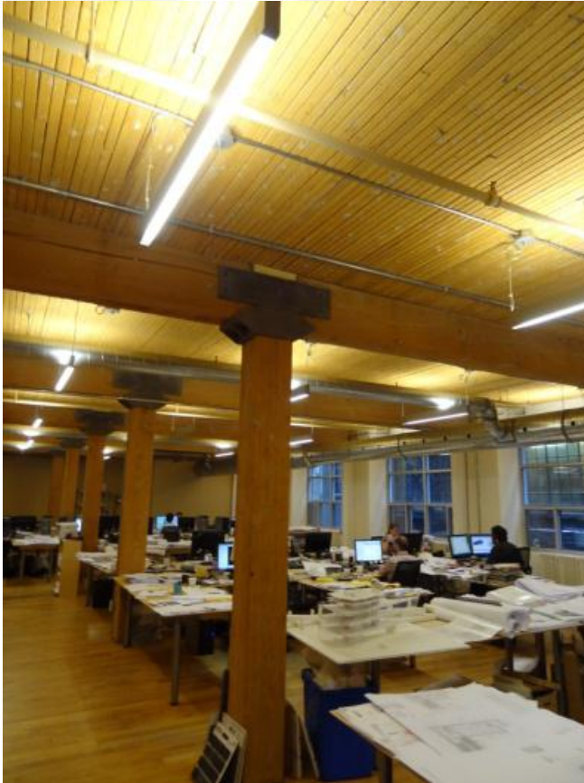
Post & Beam with wood planks
