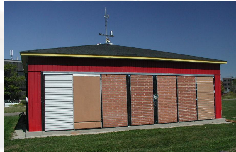
U. of Waterloo BEGhut Test Facility
